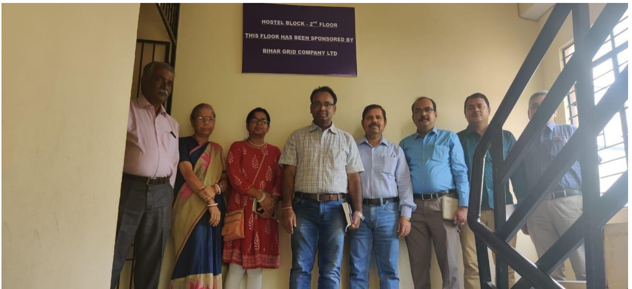
Visit of Officers of Bihar Grid Company Limited during the construction of these second floor of Hostel building of girls' free residential school Sister Nivedita Valika Vidyalaya run by NGOM/sNaiDharti
