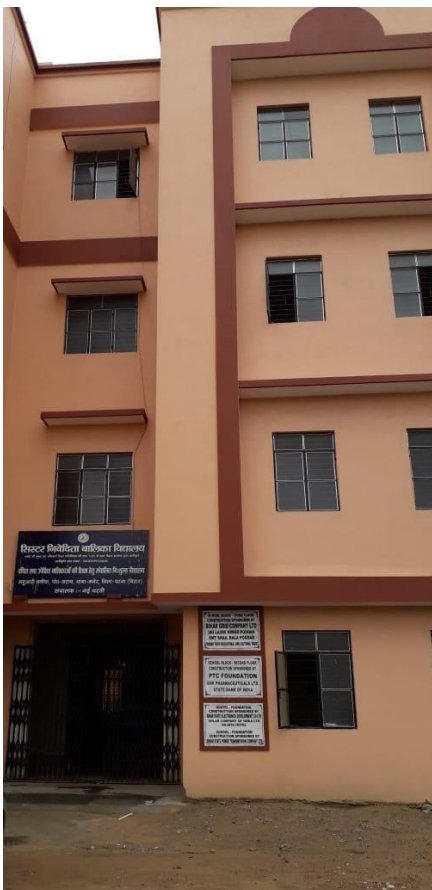
Completion of construction of third floor of School building of girls' free residential school Sister Nivedita Valika Vidyalaya run by NGO M/s Nai Dharti funded by Bihar Grid Company Limited under CSR activities of the Company
