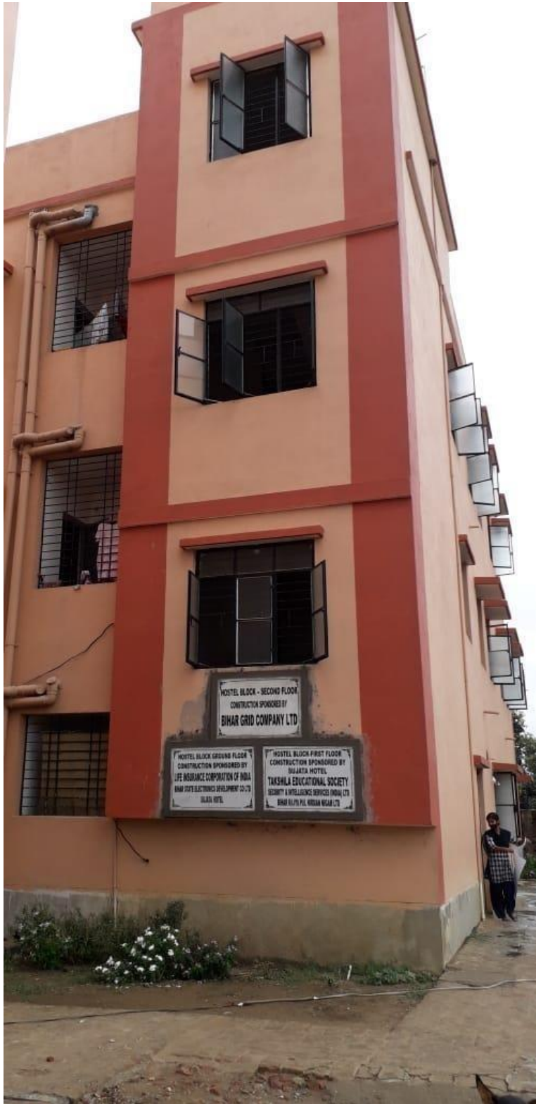
Construction of the second floor of Hostel building of girls' free residential school Sister Nivedita Valika Vidyalaya run by NGO M/s Nai Dharti completed by Bihar Grid Company Limited under past CSR activities of the Company
